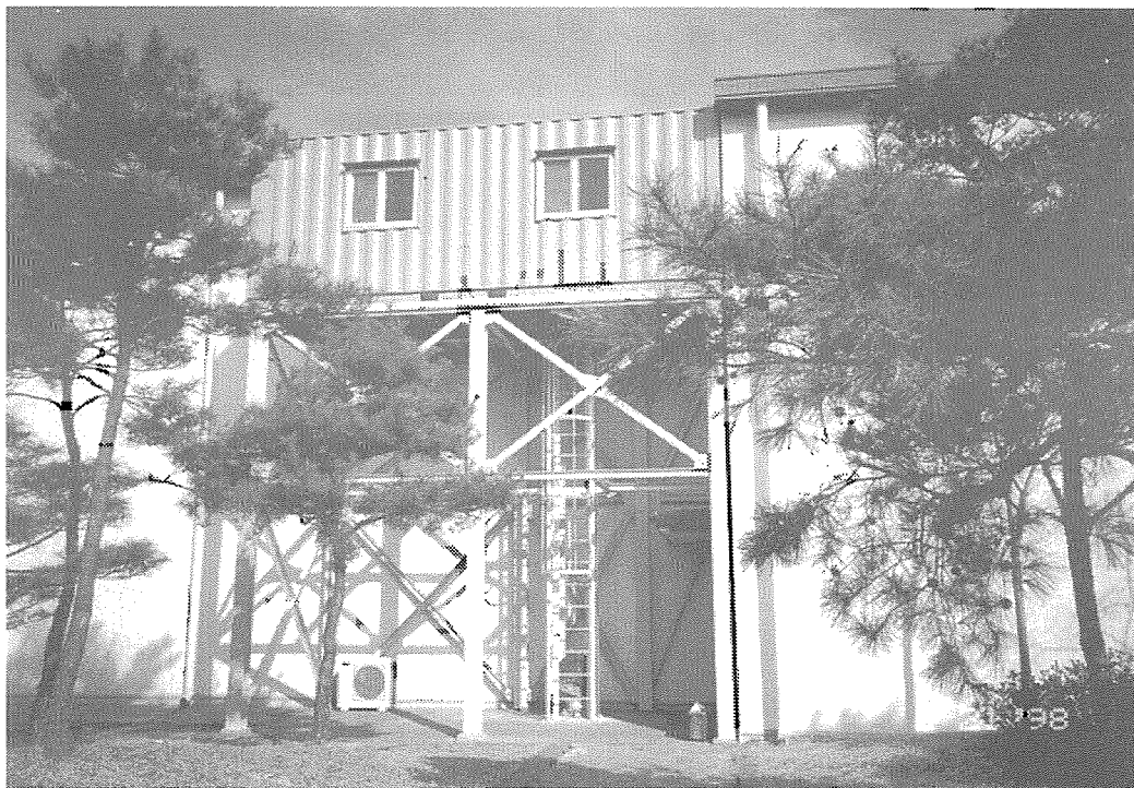
Fig. 4. Picture of constructed TOF facility
